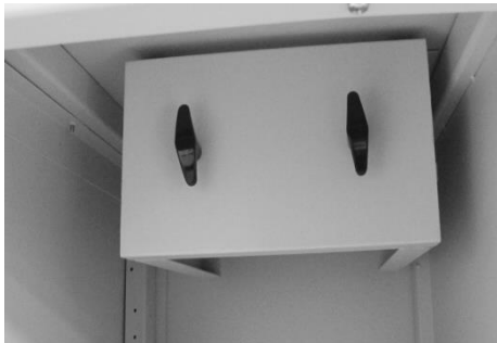
Figure 2.2. Shielded Access Door Beneath L- Shield.
